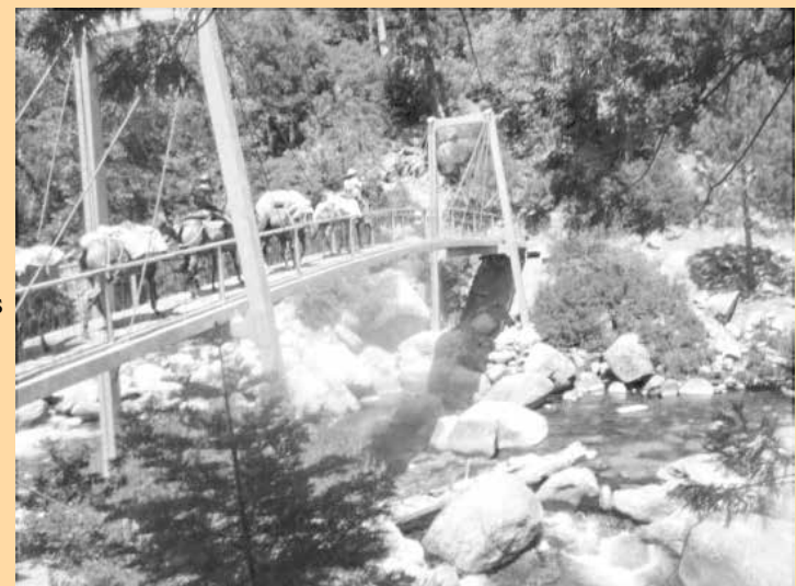
Denise and Mary with their strings on the bridge at Sheep's Crossing on the San Joaquin River
