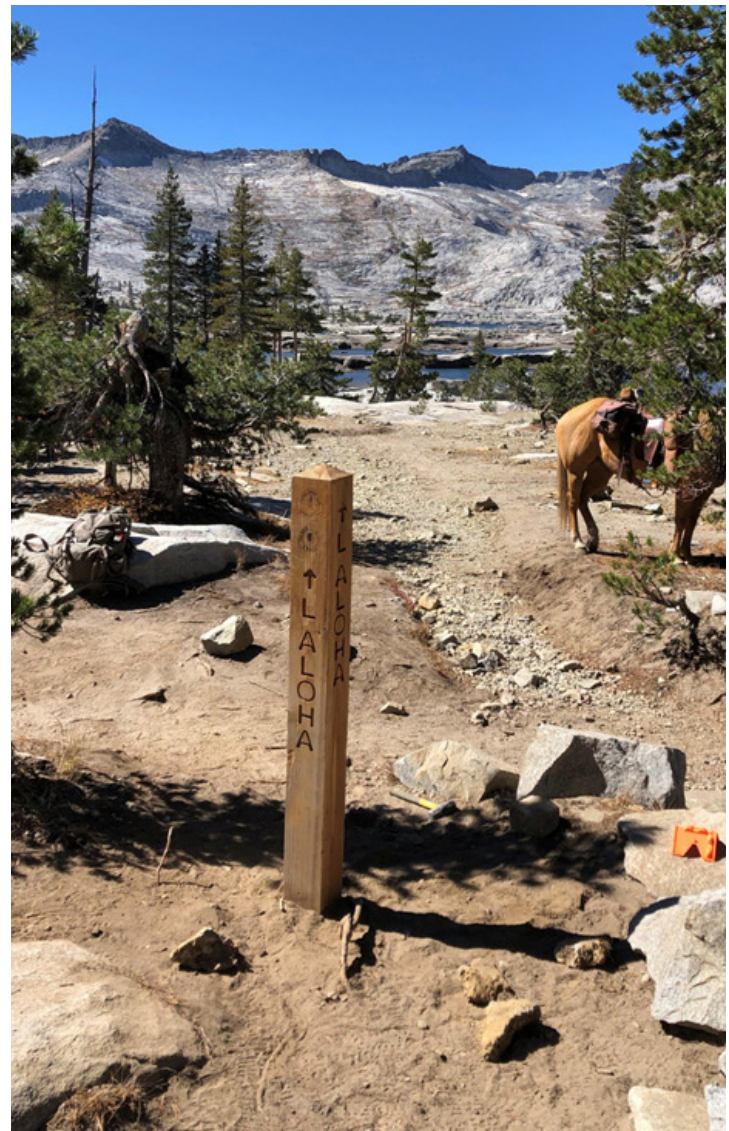
New post installed.
