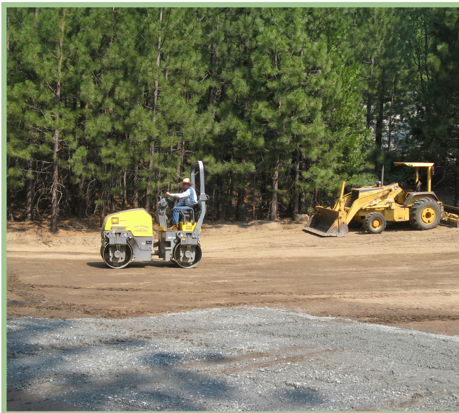
XP Corral-gravel install.
