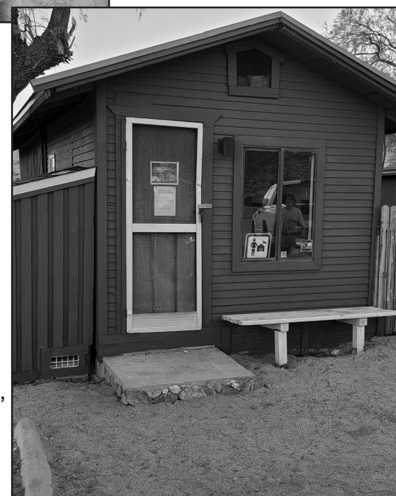
Campgrounds were cleaned, buildings repainted, roofs replaced, doors and eaves repaired.
